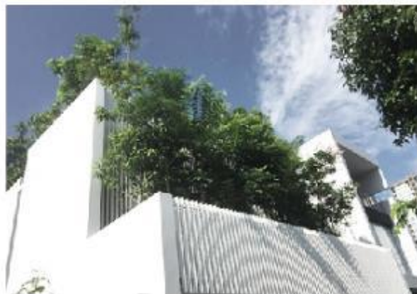
3 months after completion
