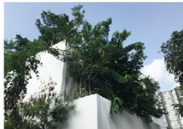
10 months after completion
