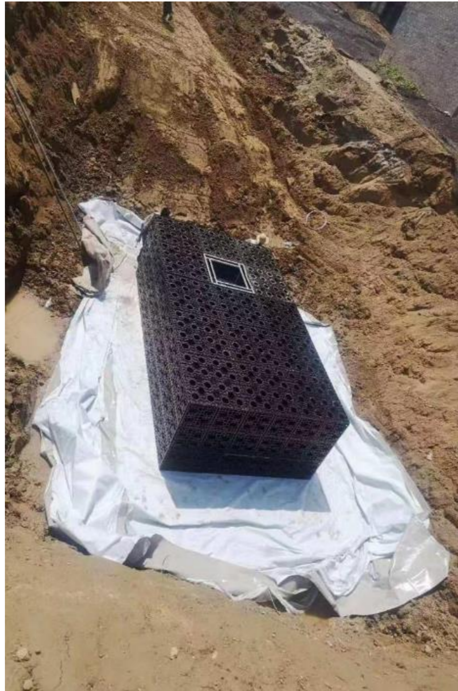
Rainwater harvesting pool construction
