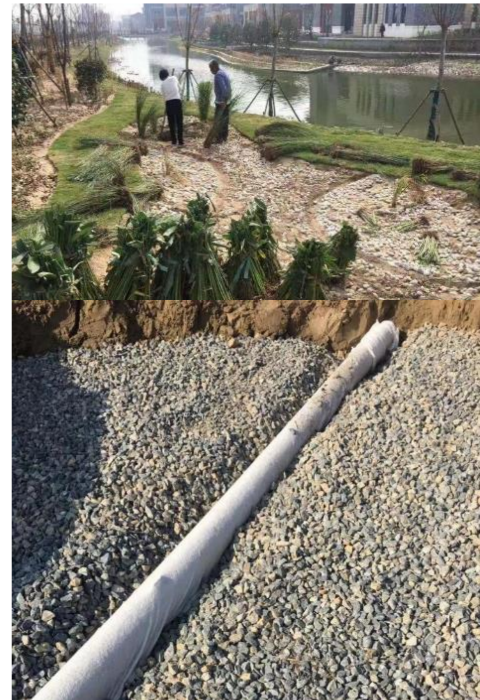
Rain garden construction
