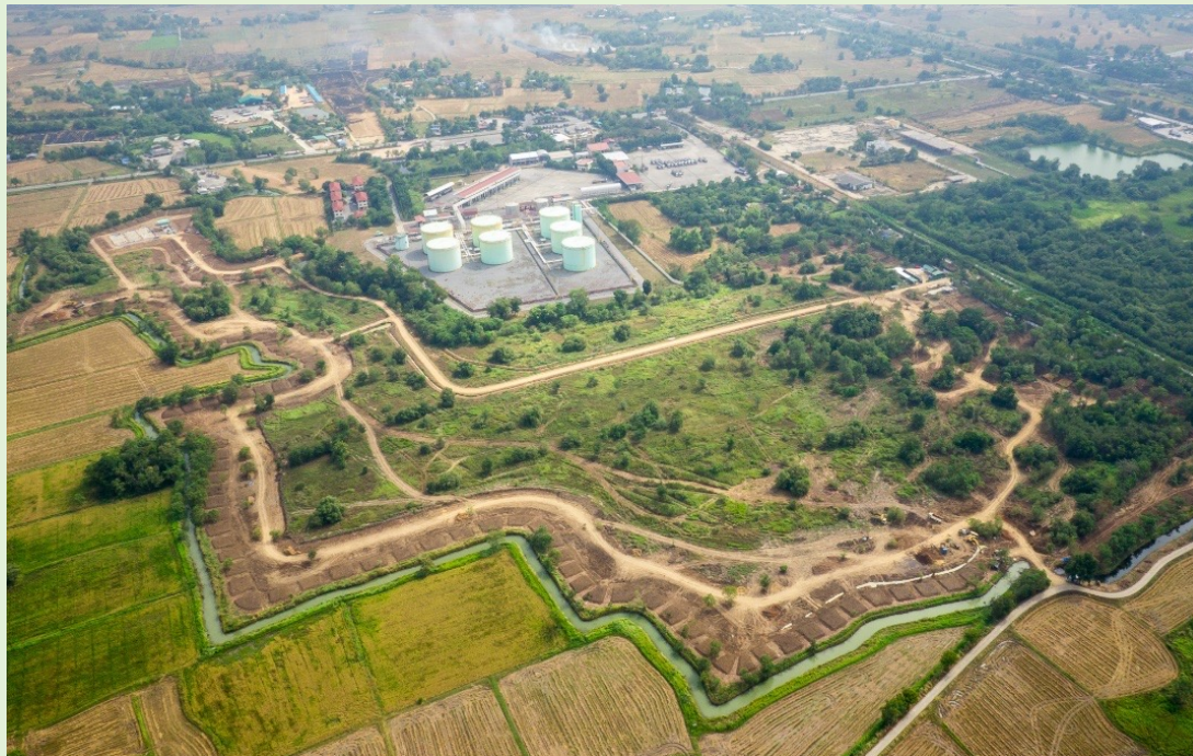
Oil Terminal Saraburi ▶
