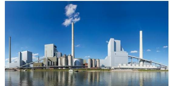
Heat Pump using the Rhine as part of „Reallabor der Energiewende“
