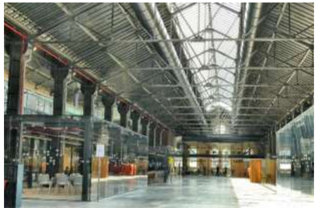
Figure 4: Internal view of OGR
